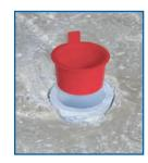
2. Insert plug to keep conduit clean/dry through balance of rough-in. Once rough-in is complete, remove plug and continue with step 3.
