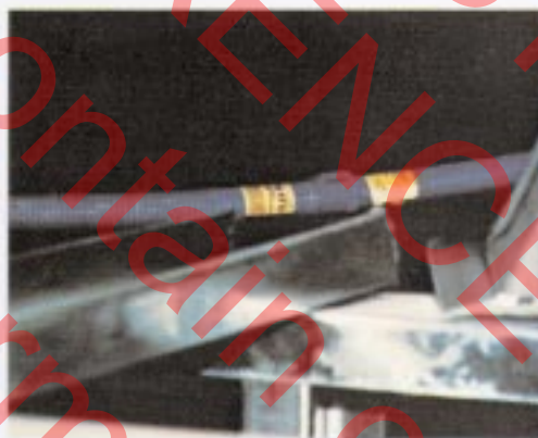
4 ENT™ running above apartment bedroom showing coupling for tubing. See Diagram II.
