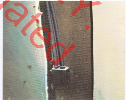
10 Outlet box shown in photo 9 from exterior of room with wall board cut away to show box and tubing still undamaged. See Diagram I.
