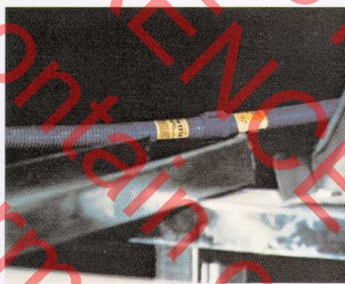
4 ENT™ running above apartment bedroom showing coupling for tubing. See Diagram II.
