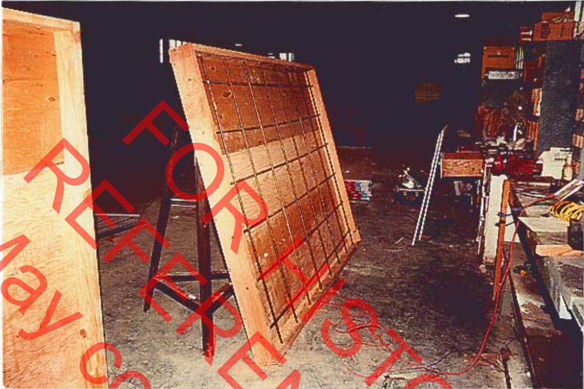
1. Rebar placed in form.
