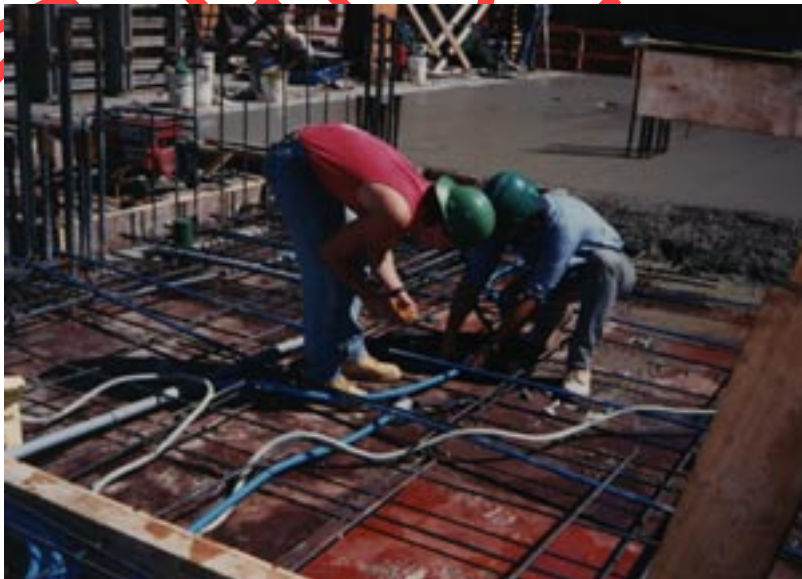
Figure 2: ENT installation in Marriott Hotel project. Cleveland, Ohio.
