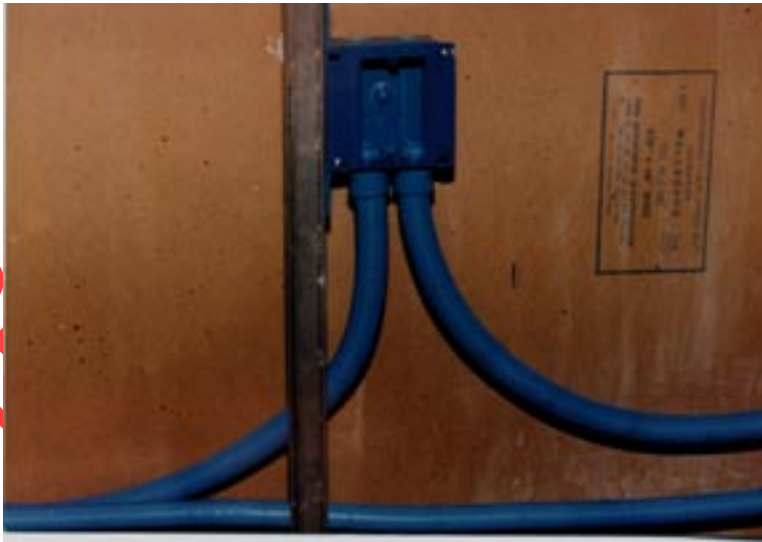
Figure 43: ASTM E-119 ENT box installation, pre-test
