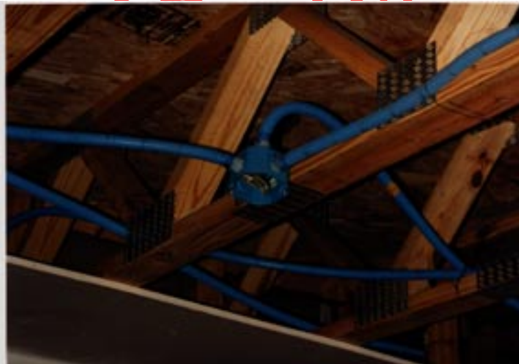
Figure 31: ENT used with pre-manufactured wood trusses
