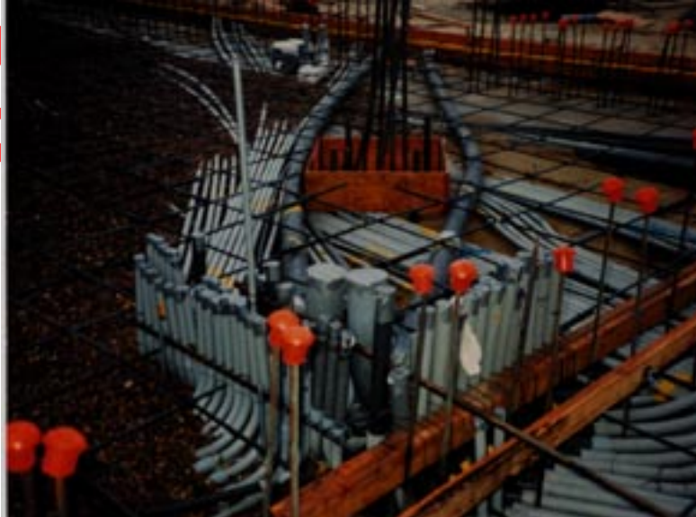
Figure 3: Use of ENT in hotel foundation application Disney World, Florida
