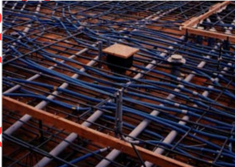
Figure 46: ENT installed in highrise hotel-Four Seasons, La Jolla, California
