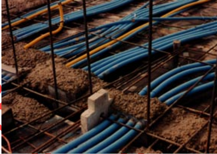
Figure 38: Use of ENT in concrete slab application
