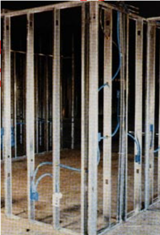
Figure 6: ENT use in steel stud partitions
