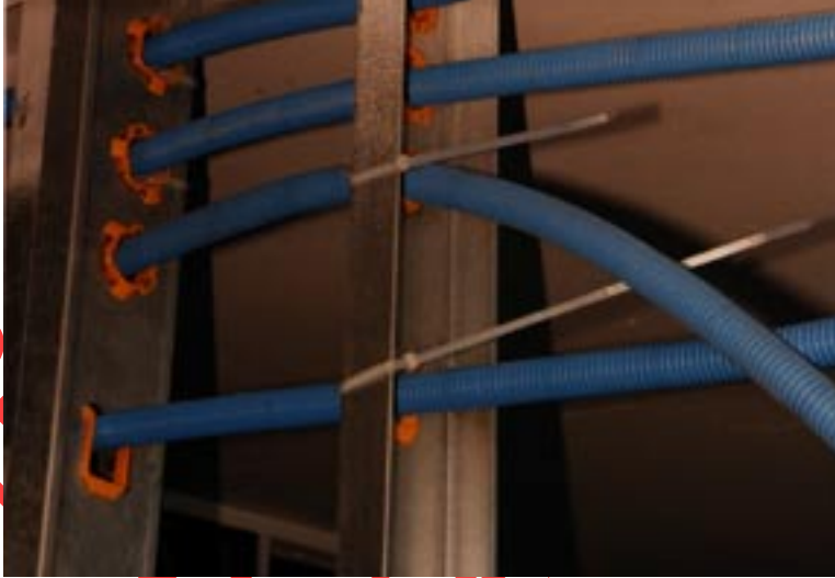
Figure 28: Metal studs with bushings installed Disney World, Florida
