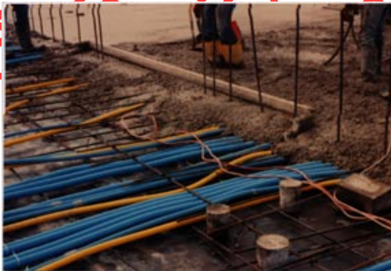
Figure 33: ENT installed in concrete slab Key West, Florida
