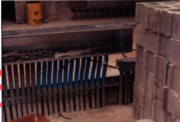
Figure 30: ENT riser to trough Key West, Florida
