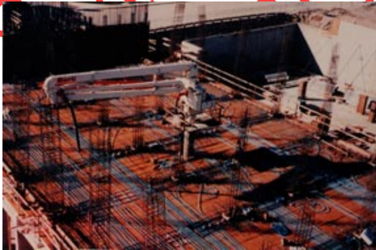
Figure 49: Street level view of ENT being installed in highrise structure, Southern California
