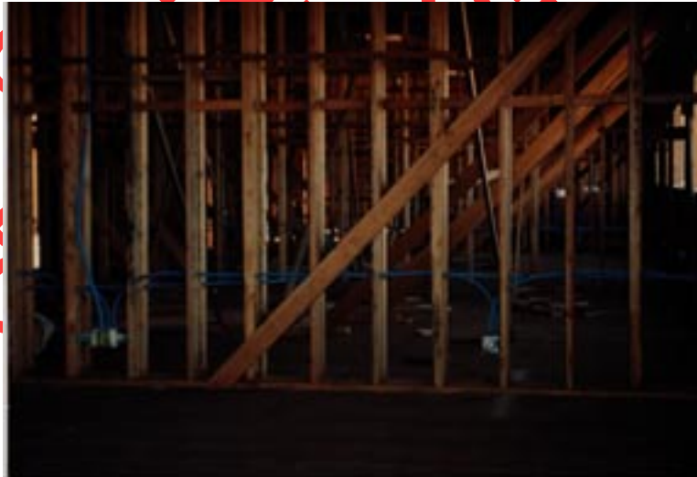
Figure 29: ENT installation in walls of Type V building Kissimee, Florida
