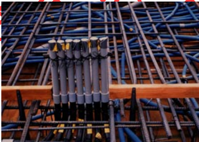
Figure 45: ENT installed prior to concrete pour in highrise structure, Southern California
