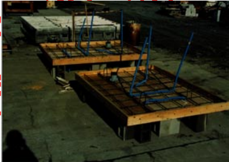
Figure 37:Preparation of 2-hour ASTM E-119 test slabs
