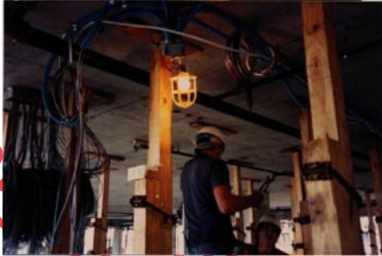
Figure 25: Installation of ENT in Type I Building Disney World, Florida
