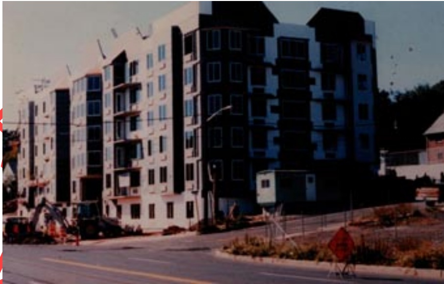
Figure 4: Highrise apartment complex utilizing ENT. Patterson, New Jersey
