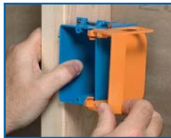
2. Clip the Add-On Bracket onto the edge of the electrical box.
