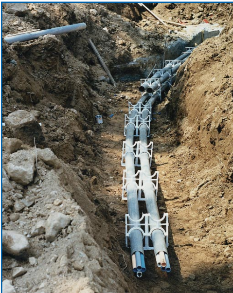
Pulled through existing conduits
