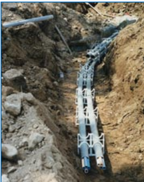
Pulled through existing conduits
