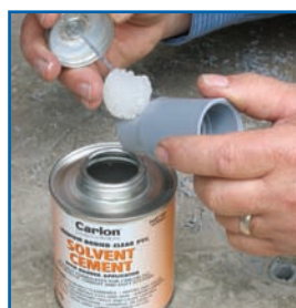
Apply a uniform coat of cement.
