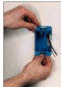
Place Box in Wall
