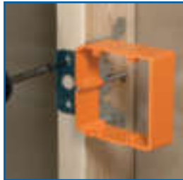
2-Gang Adjustable Low Voltage Bracket SC200ADJC
