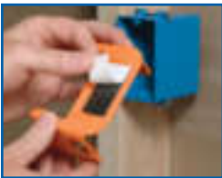
1. Pull the adhesive tape tab.
