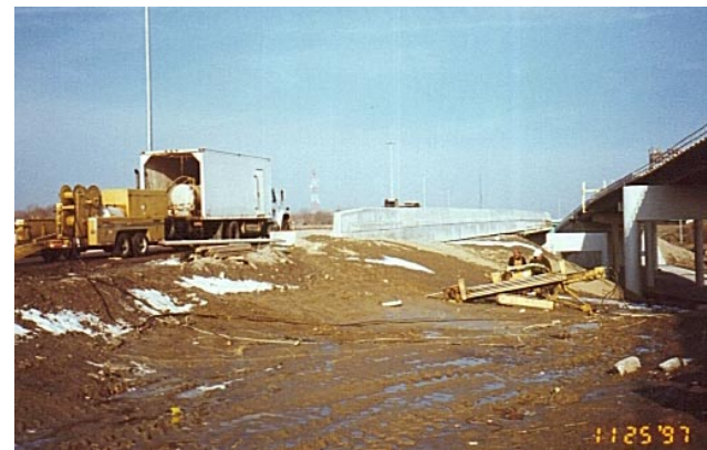
Above Left: The 8 inch diameter reamer is seen here along with the strain gauge and on-board computer used to measure the pull force on the pipe. An expandable pulling eye was used to grip the leading end of the pipe. Above Right: The directional boring machine and a 1,200 gallon water tank.
