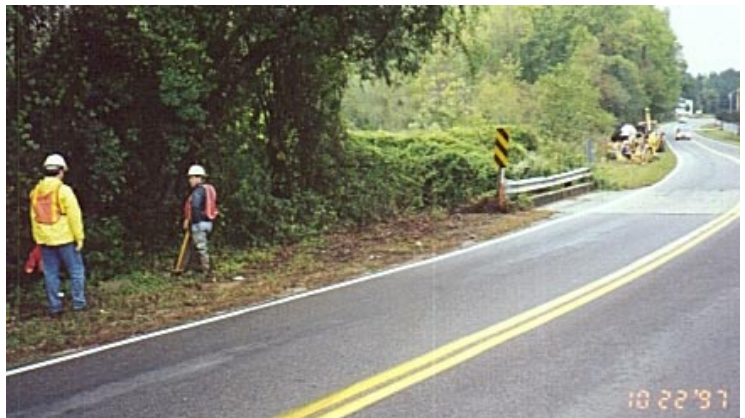
Left: Facing the drilling rig (top left) overlooking the creek. Directional drilling and Bore-Gard pipe was the least cost option for this varied-terrain 180 ft. bore. Trenching was not an option. Above Right: A look at the 180 ft. span of the bore from far left to far right (drill rig) of the picture.
