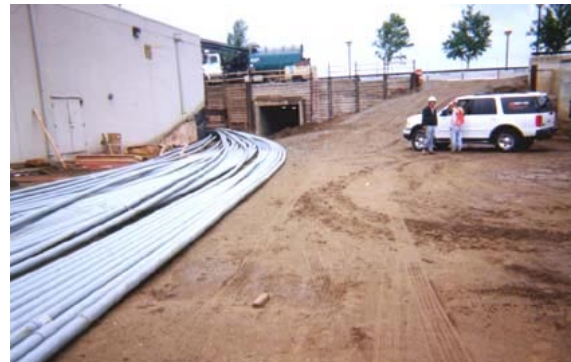
Above Left: A 200 ft. bore under a canal and roadway was needed to connect the Indiana State Museum with the new Administration Building. Above Right: Carlon Bore-Gard has a 65 degree bend radius making it flexible enough to be pulled around a building.
