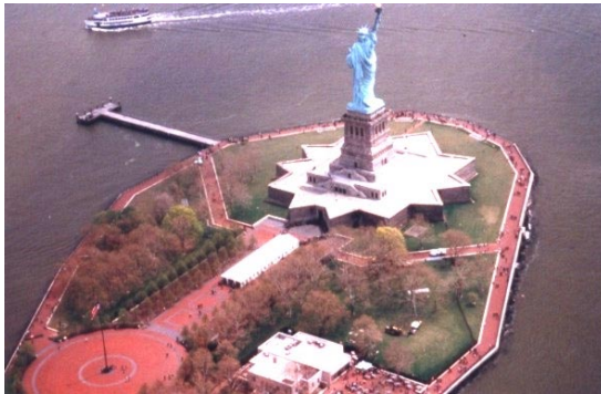
Left: Limited spaces and minimizing disruption to the pristine environment and daily tourist activities made Horizontal Directional Drilling and Carlon Bore-Gard the ideal solution.
