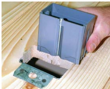
Install clip over subfloor.
